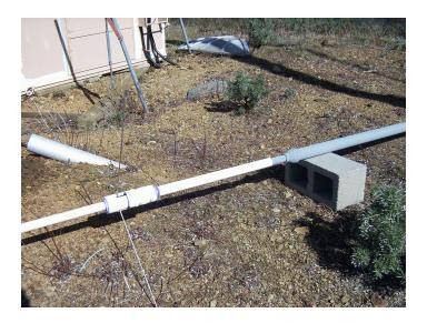
There's the final assembly-the 1" base mount pipe threaded into an adapter to the 2" pipe mast. The PVC armor now extends down nearly three feet over the pipe-this should provide enough leverage so it won't need to be guyed farther up.
