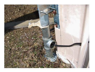
The coax doesn't see the light of day until it exits the inside of the mast near the ground.
